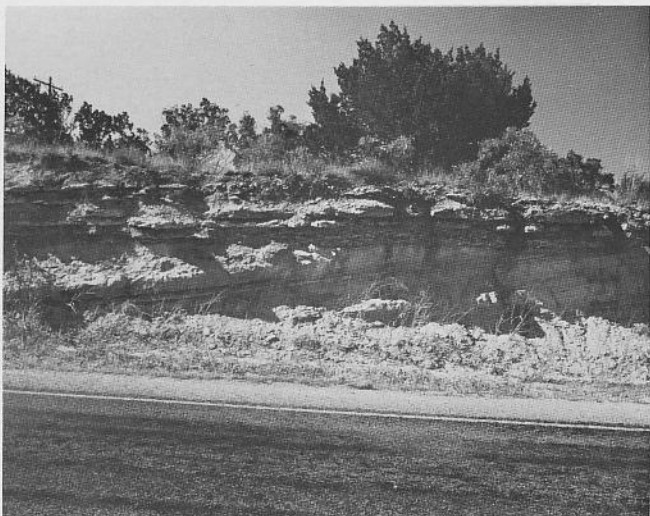
Fig. 28. Locality 45. The Lake Merritt Member, the basal portion of the Paluxy Formation in Area Six, consists of alternating sand and clay beds that exhibit sedimentary structures of large- and small-scale, low-angle planar cross-bed sets with angles of inclination ranging from 20 to 45 degrees. The angular beds of the Lake Merritt Member are overlain by horizontal beds of the Bull Creek Member of the Walnut Formation.
