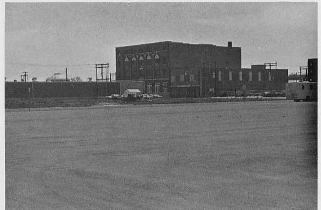
Fig. 35. Large buildings block flood flow in the flood plain. This causes increased velocities and higher stages.
