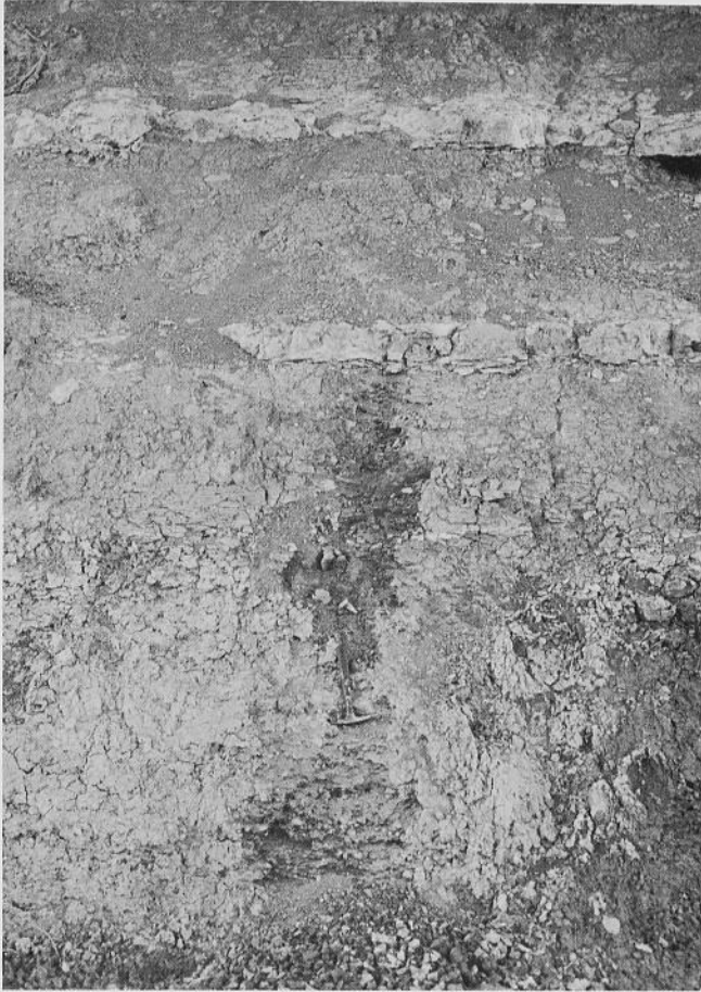
Fig. 38. View of Hill's section 8 near his "first cut" on the Missouri and Pacific Railway showing a portion of B and C, Gryphaea breccia and "friable yellow limestone." This exposure is beneath a bridge over the railroad switching yards in downtown Fort Worth. Hill, 1886a, p. 25.
