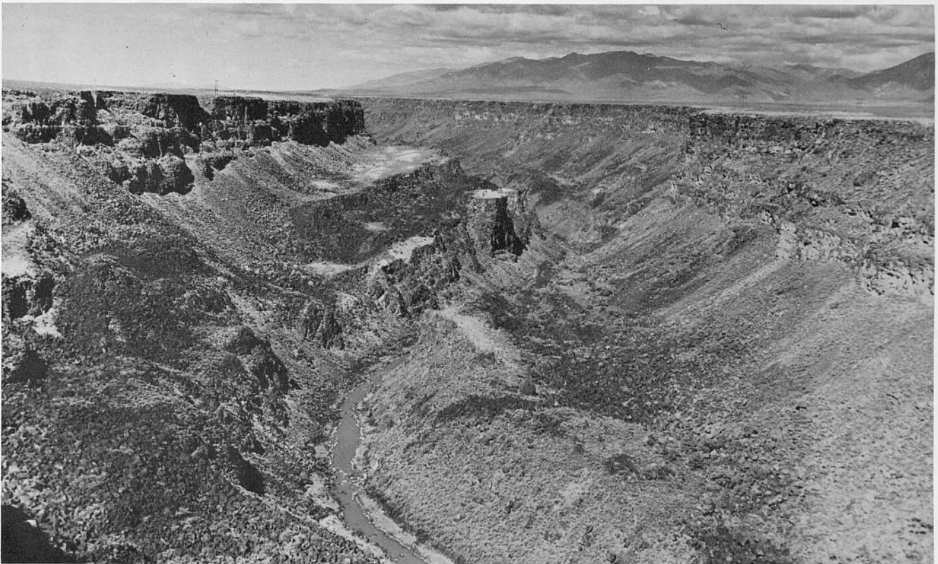
Fig. 15. (Locality 120) Slump blocks in the Rio Grande Gorge have widened the canyon. Note that the alluvial cover atop the slump blocks is similar to that atop the canyon walls.
