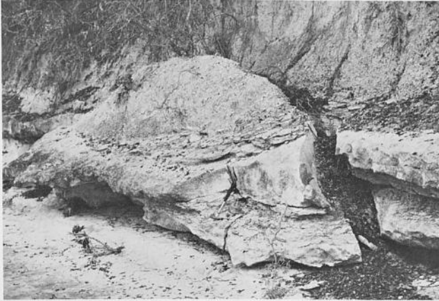
Fig. 8. Rockfalls are common in the "lower" Austin Chalk (Loc. 11), where bentonite seams are present. Here a major block of chalk has failed along joint planes. Knowledge of the local geologic section will aid in anticipating such problems.
